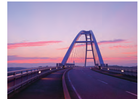
the Shima ohashi Bridge 志摩大橋
