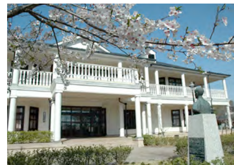
Ozaki Gakudo Memorial House 尾崎鸞堂記念館
